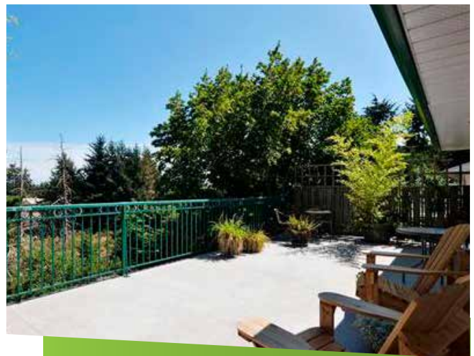
Above: Exterior views of Haida House
